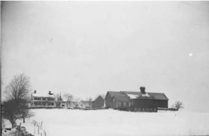
DSC03230 Charles F. Dodge Farm c 1895 This house with attached barns remains very much the same on Tucker Mill Rd. The house is now apartments. Today it is known as the Welch Farm.
