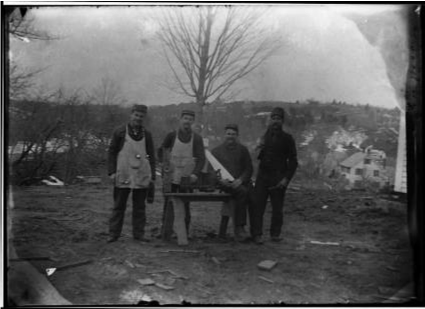
DSC02943 This is entitled "Uncle Edd and the Boys" It's not clear which one is Uncle Edd, but it seems that they're at work putting the finishing touches on the Atwoods' Prospect Cottage.
