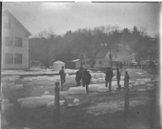
DSC03242 :Late winter always brings flooding associated with ice floes melting and breaking up. This shows an unusually severe example where the ice and water came up to Dodge’s steps.
